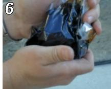
Open Eli-Flex FR909 kit, remove the spine and mix the two components together for 2-3 minutes or until warm. See "Six Easy Steps to Belt Repair" for more detailed instructions.
