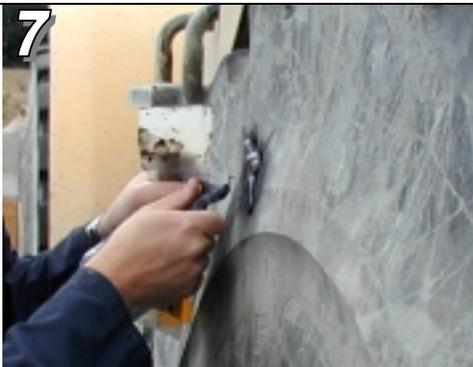
7 Cut open a corner of the bag and apply a liberal amount to the center of the gouge. You have 20-30 minutes of working time.
