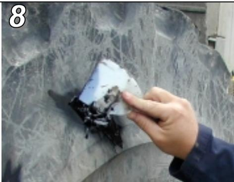
8 Use your spatula to force the Eli-Flex into the gaps by working from the center outwards. This will help reduce air entrapment and bubbles forming.
